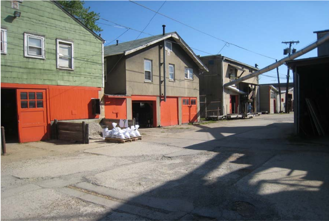
Storage Buildings (Could Be Removed For Outside Storage)
