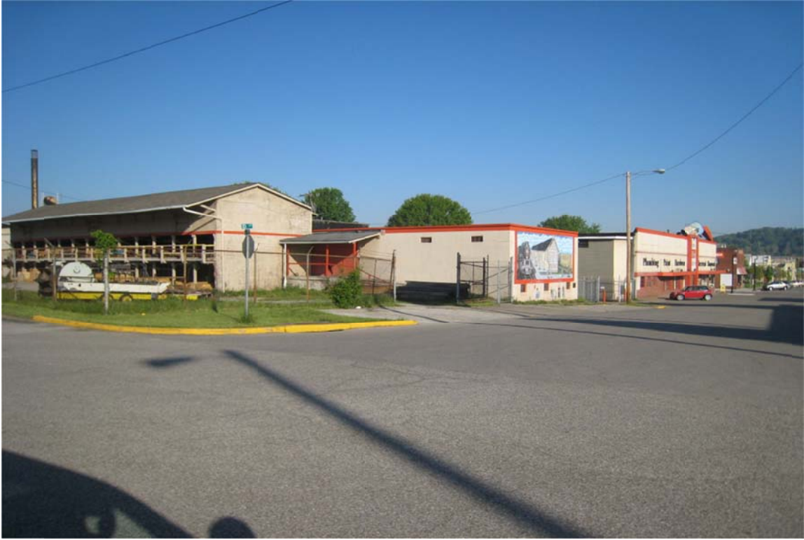
Lumber Sheds (View From D Street & 1 st Avenue)
