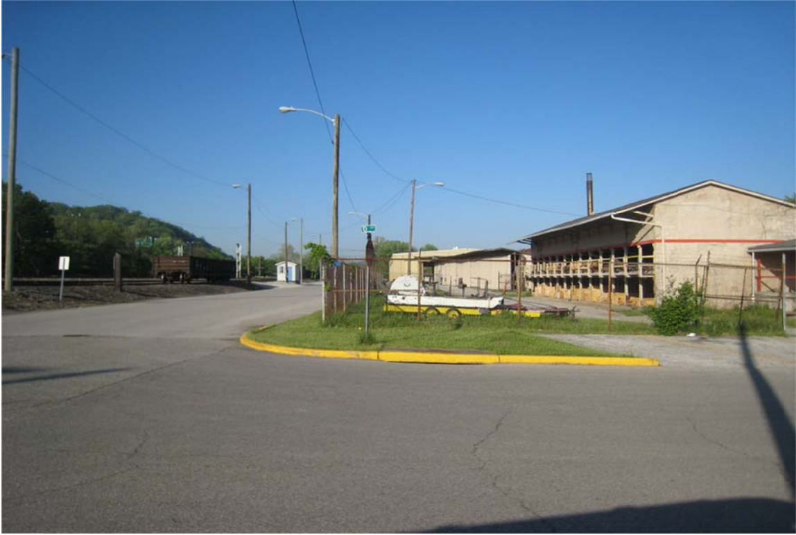
Lumber Sheds (1 st Avenue Looking West)
